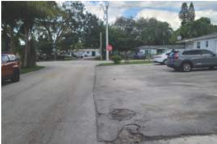
Existing asphalt parking area in location of future sidewalk
