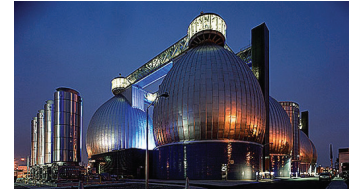
Newtown Creek Wastewater Treatment Plant 2014 ACEC National Recognition Award
