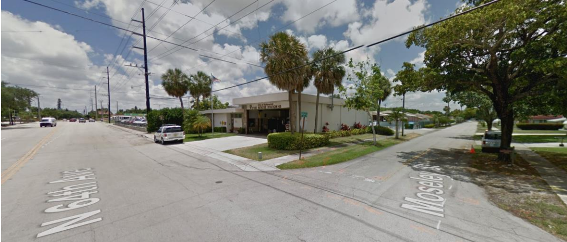
View of Property and Adjacent Structures, Looking South-West
