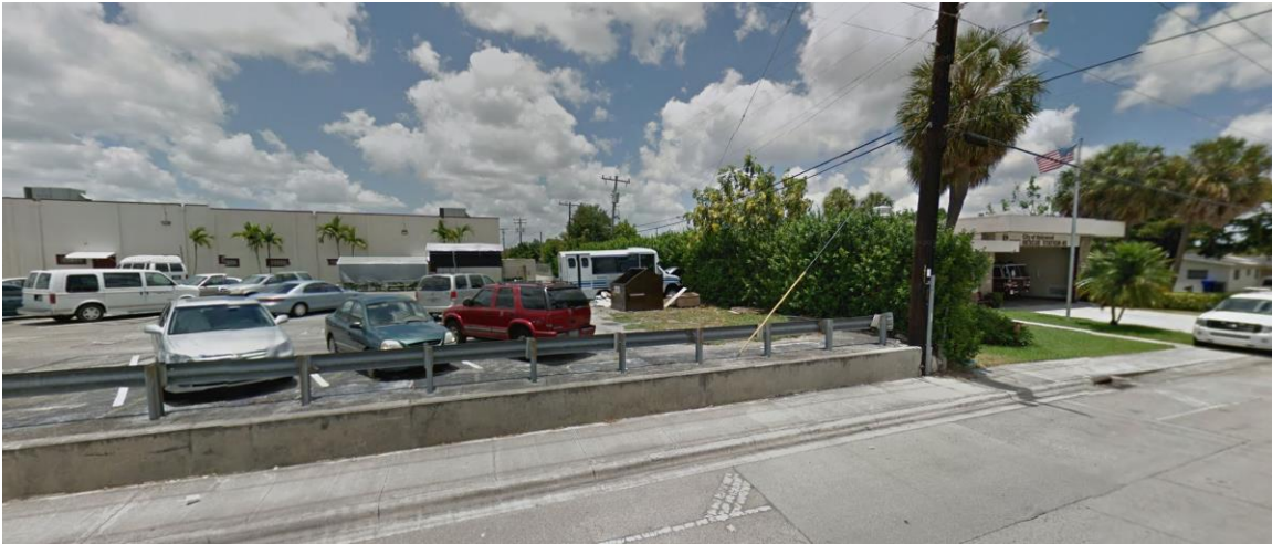
View of Property and Adjacent Structure, Looking West
