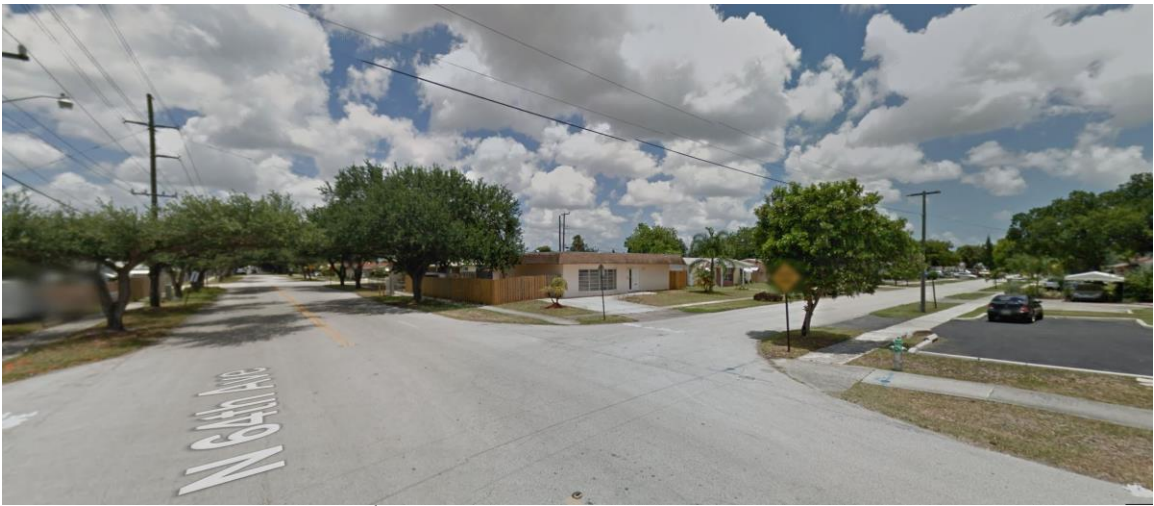
Adjacent Structure across N 64 th Avenue, Looking North-East
