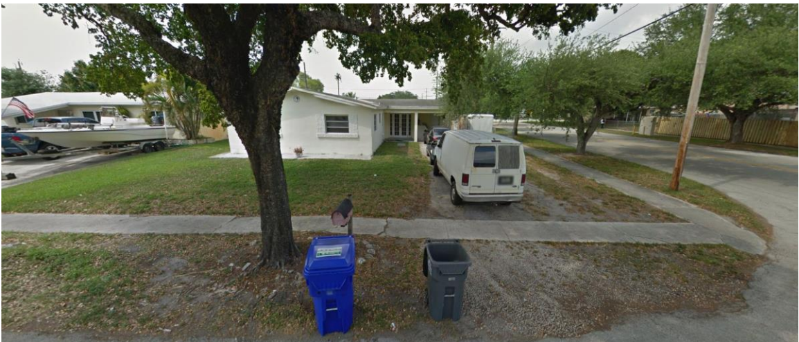
Adjacent Structure across Mosley Street, Looking North
