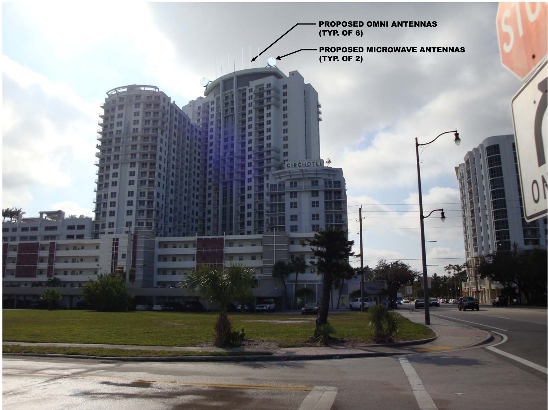
MOTOROLA SOLUTIONS CIRC HOTEL - ROOF MOUNTED ANTENNAS VIEW 1 - VIEW FROM THE NORTH (BROWARD COUNTY)
