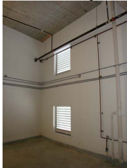
Vents near wall penetration location
