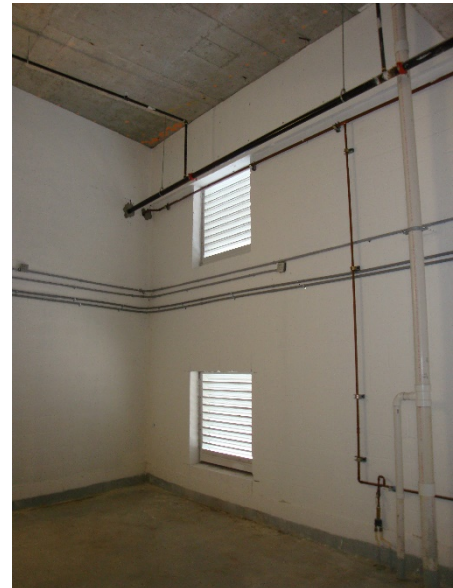
Vents near wall penetration location
