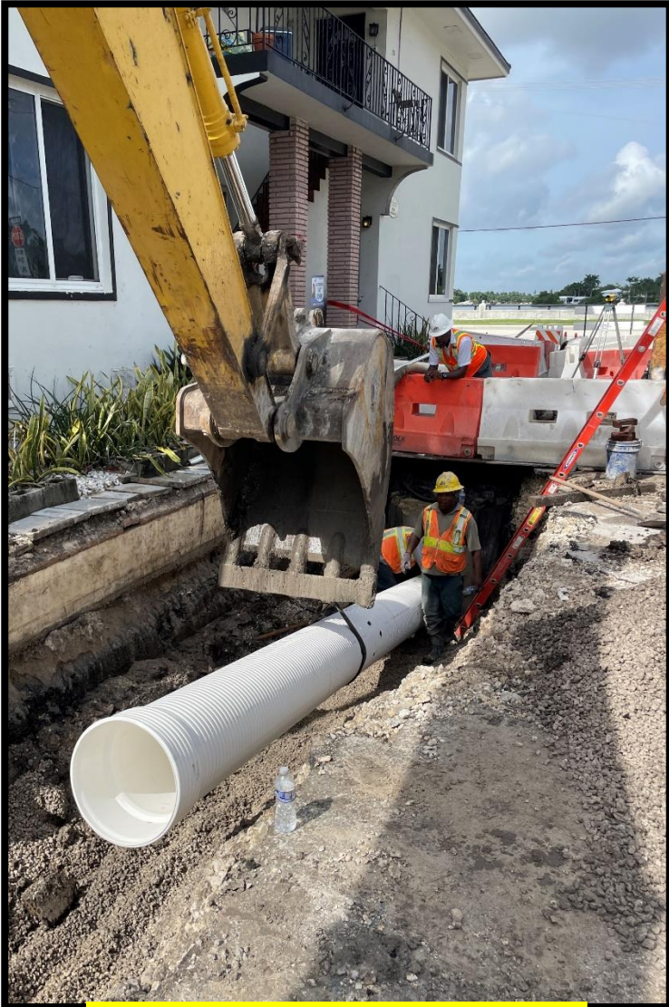
Stormwater pipe installation
