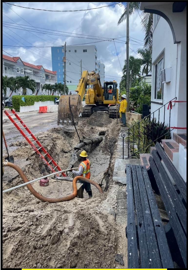
Excavation for pipe installation
