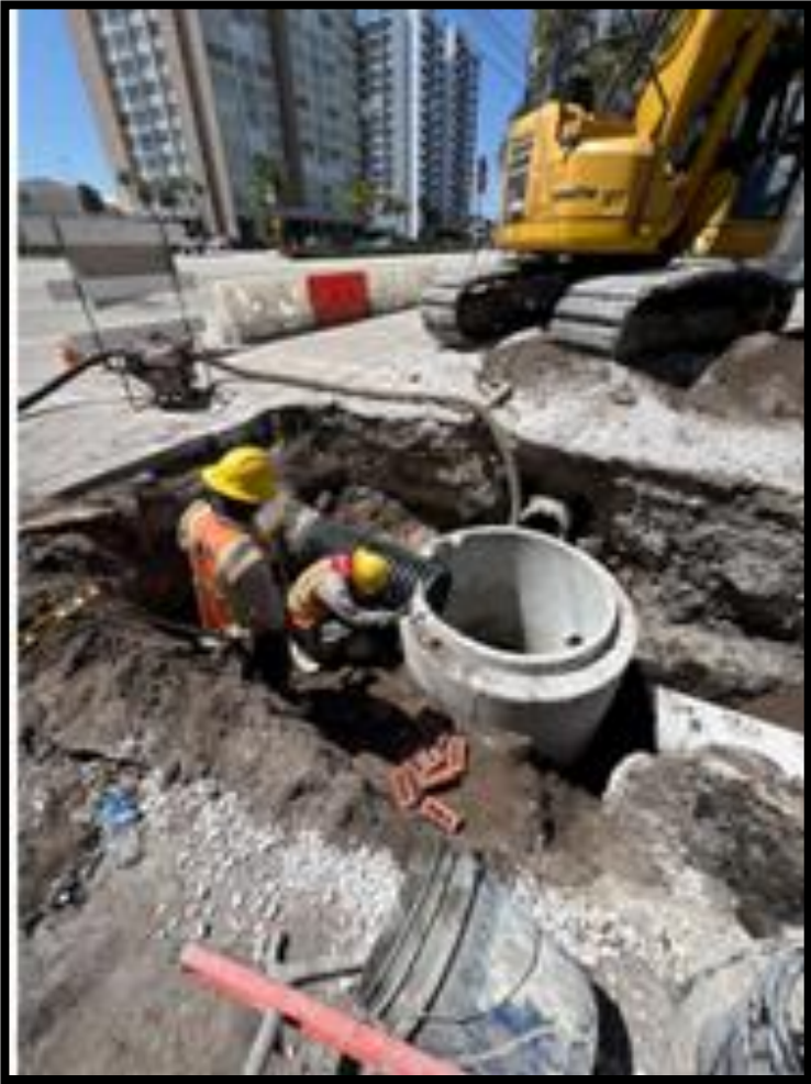
Drainage Structure Installation
