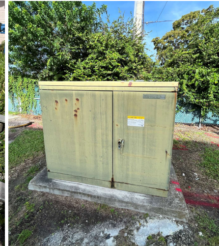
Figure A-4: Abandoned FPL Transformer
