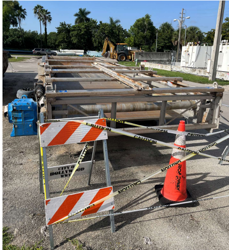
Figure A-2: East Bar Screen Removed from Service
