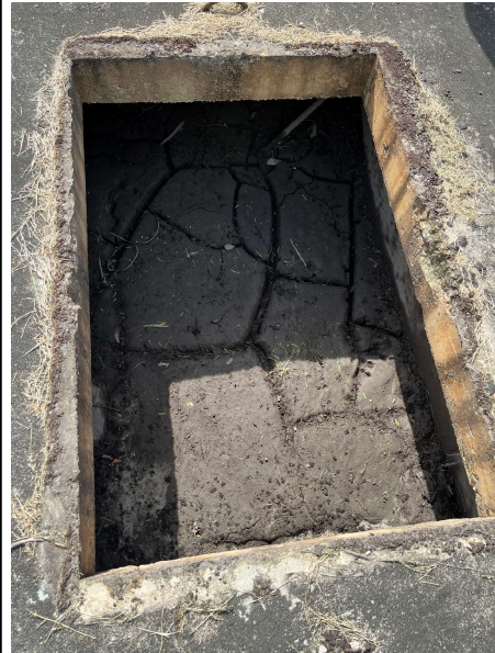
Figure A-6: 5.3'x7.0' Electrical Vault
