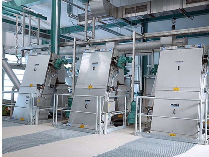
Figure 3-1: HUBER Technology RakeMax Bar Screen
