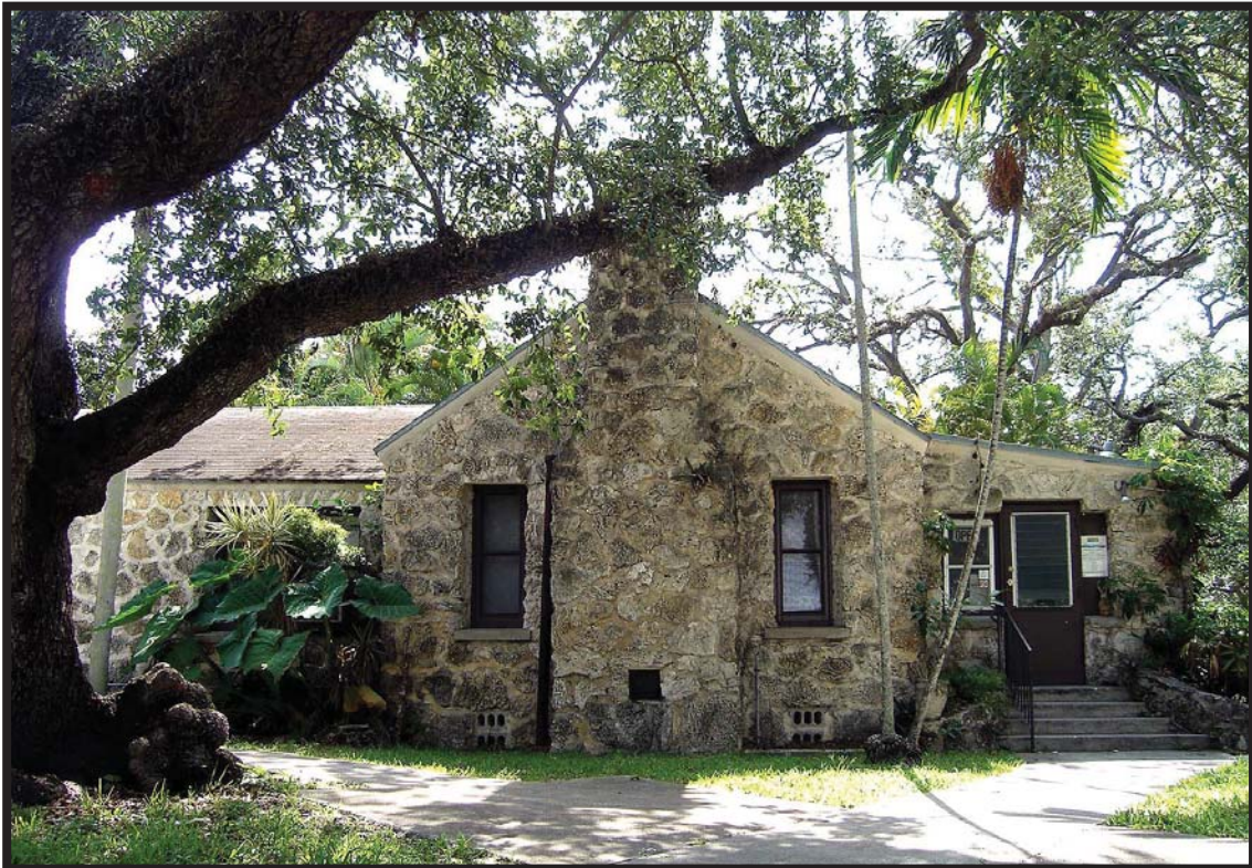
Photo #1 - Butler Rock House West Façade, Prominent Exterior Gable Fireplace, Entrance to enclosed porch, Oolitic Limestone finish, looking east
