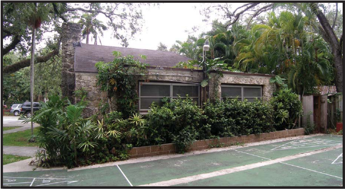
Photo 3 – Butler Rock House, West and South Facades, looking northeast. Building profile, prominent gable chimney and entrance to the enclosed screened-in porch and 4-step platform entry, looking northeast.
