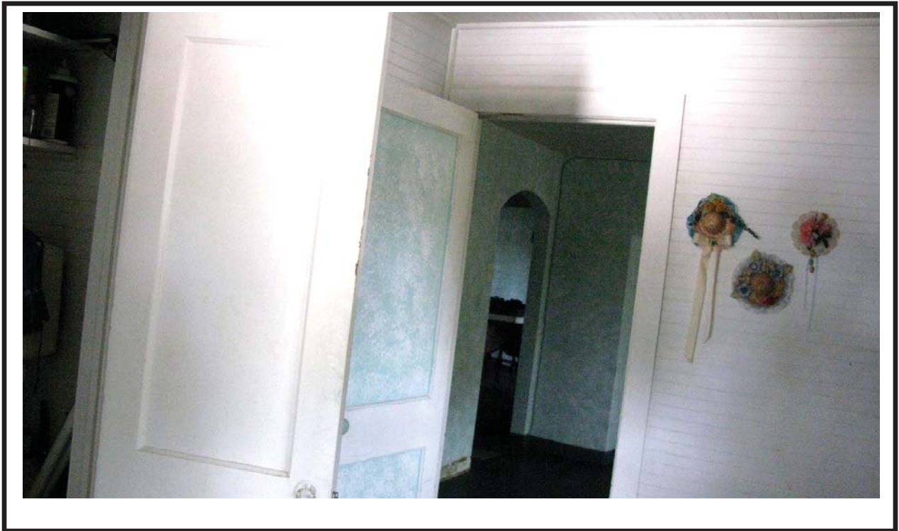
Photo 5 - Butler Rock House Interior showing solid double-panel wood door, bead board wall and one of many segmental arched opening.
