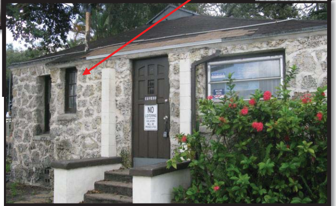
Photo 4B – Butler Rock House partial North Façade with Clipped gable roof, 4-step platform entry, masonry stringer, single wood panel door, looking southeast. Original multi-pane casement window on east side of entry.
