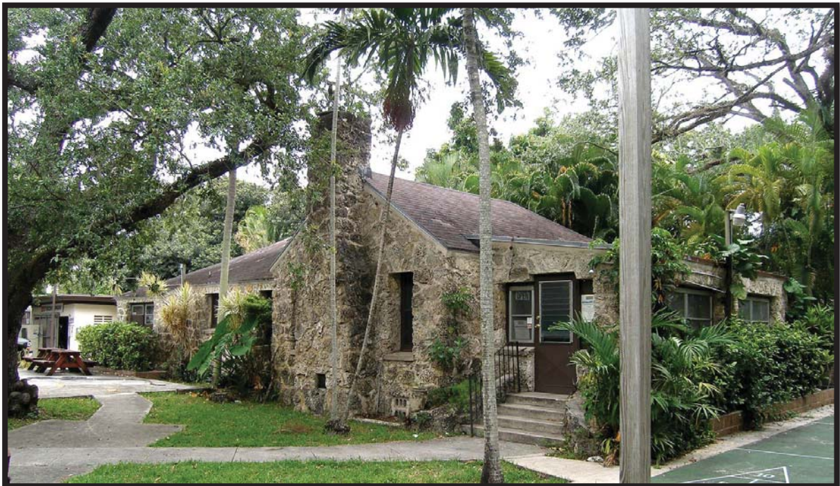
Photo # 2 – Butler Rock House, West and South Facades, looking northeast. Building profile, prominent gable chimney and entrance to the enclosed screened-in porch and 4-step platform entry, looking northeast.
