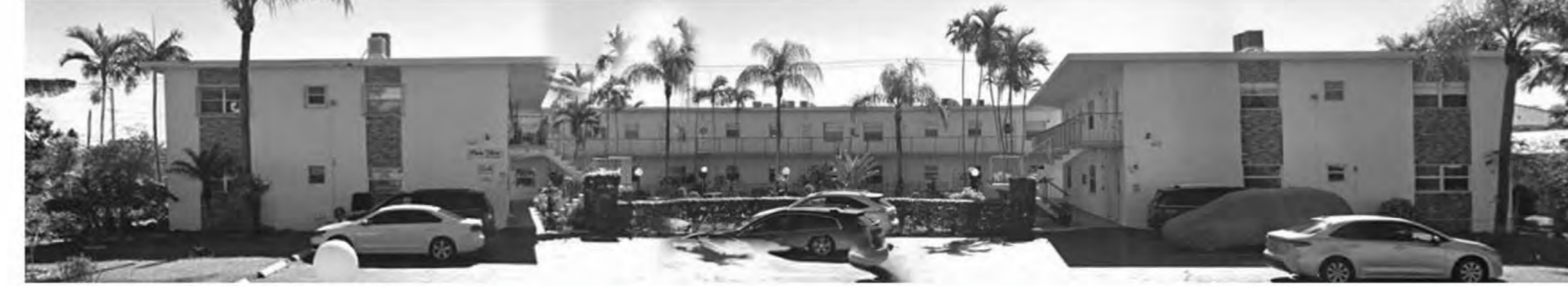
EXISTING 2240 JOHNSON St
