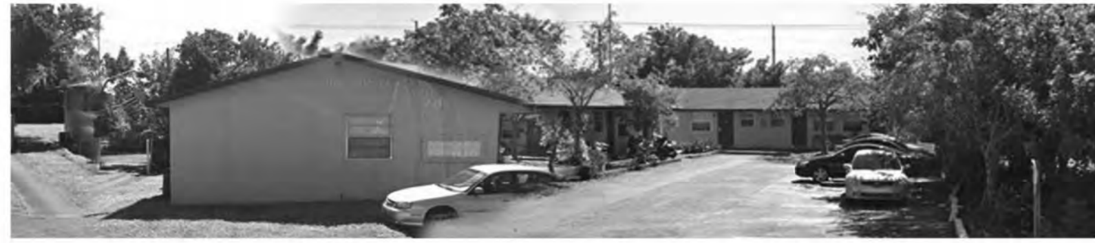
EXISTING 2216 JOHNSON St
