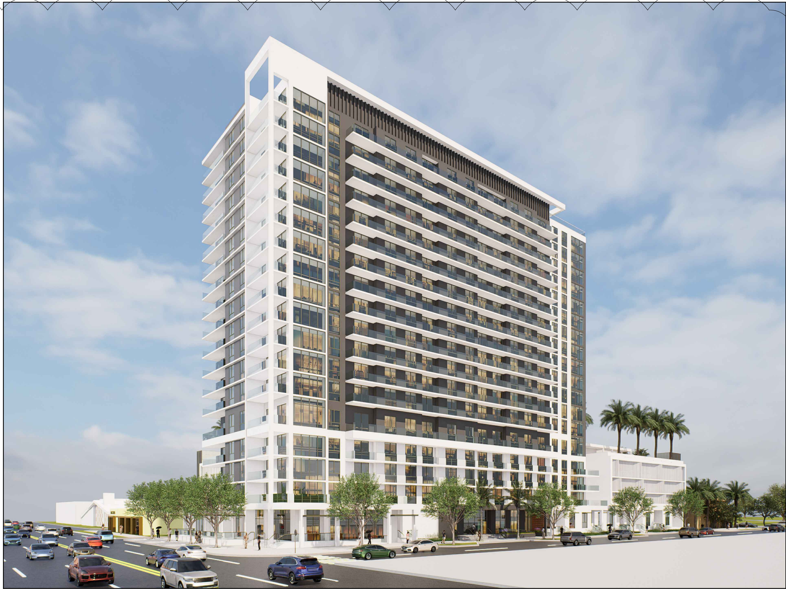
VIEW LOOKING NORTHEAST FROM FEDERAL HWY
