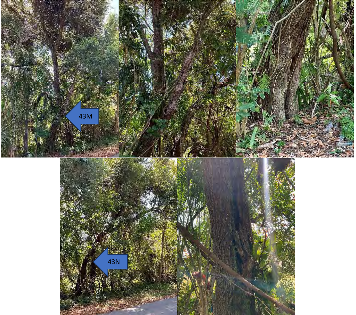
Live Oaks ( Quercus virginiana ), facing east. Note Poor structure, visual evidence of decay, storm damage, large trunk wound for Tree # 43M, and poor structure, visual evidence of decay, canopy crowding, and deadwood for Tree # 43N.
