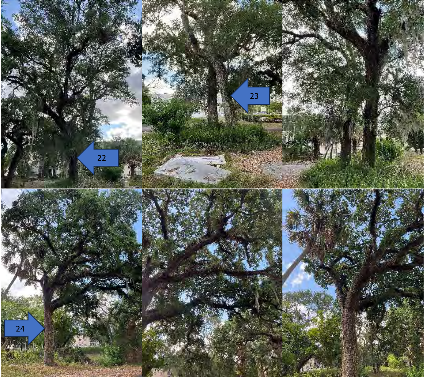
Live Oaks ( Quercus virginiana ), facing east. Note poor structure, canopy crowding, confined root space, trunk lean, deadwood, canopy dieback for Tree #'s 22 & 23. Note poor structure, unbalanced crown, deadwood, and canopy dieback for Tree # 24.
