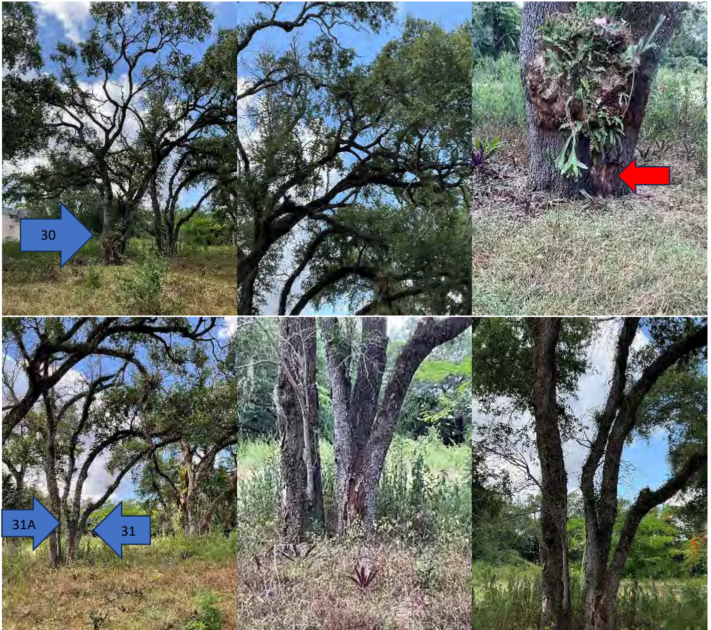
Live Oaks ( Quercus virginiana ), facing south. Note Poor structure, large diameter deadwood, canopy dieback, visual evidence of decay (red arrow) for Tree # 30. Note poor structure, canopy crowding, bark loss, visual evidence of decay for Tree # 30, and significant canopy dieback, significant deadwood, poor vigor for Tree # 30A.
