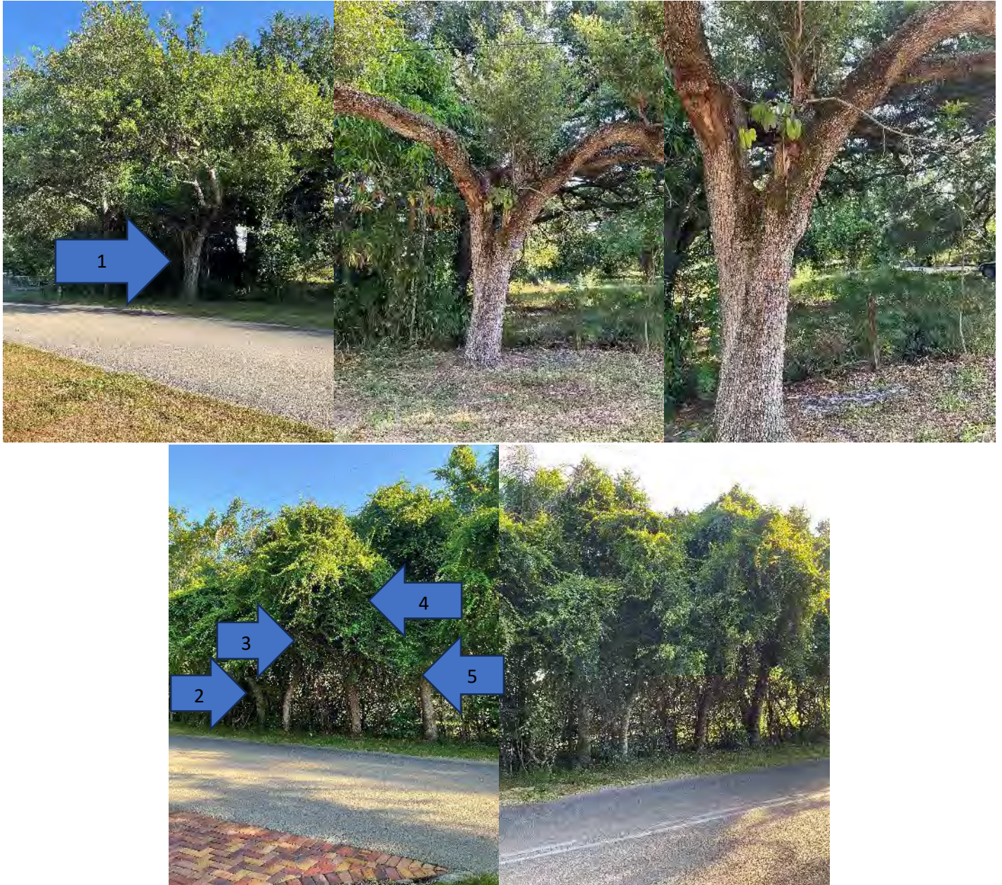
Live Oaks ( Quercus virginiana ), facing north. Note poor structure, utility pruned, water sprouts, visual evidence of decay, and deadwood for Tree # One. Note poor structure, canopy crowding, vines, visual evidence of decay, and trunk leans for Tree #'s Two, Three, Four & Five.
