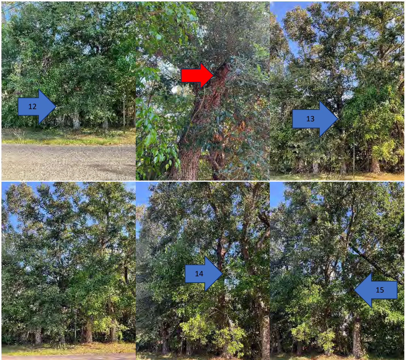
Live Oaks ( Quercus virginiana ), facing north and west. Note Poor structure, heading cuts, canopy crowding, storm damage (red arrow), for Tree # 12, and Poor structure, canopy crowding, canopy dieback for Tree #'s 13 & 14. Note poor structure, canopy crowding, canopy dieback, and utility pruning for Tree # 15.
