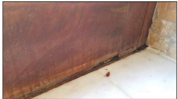
Water and termite damage to doors.
