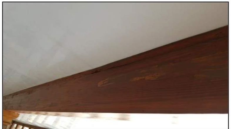
Termite damage to ceiling truss
