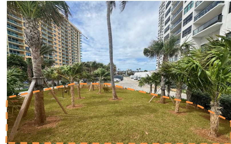
From Plumbing Chase Looking West
