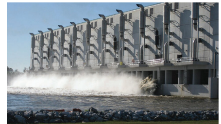
Arcadis with our construction partner, provided the design and construction of the world’s largest water management pump station, the Gulf Intracoastal Waterway Closure Complex.
