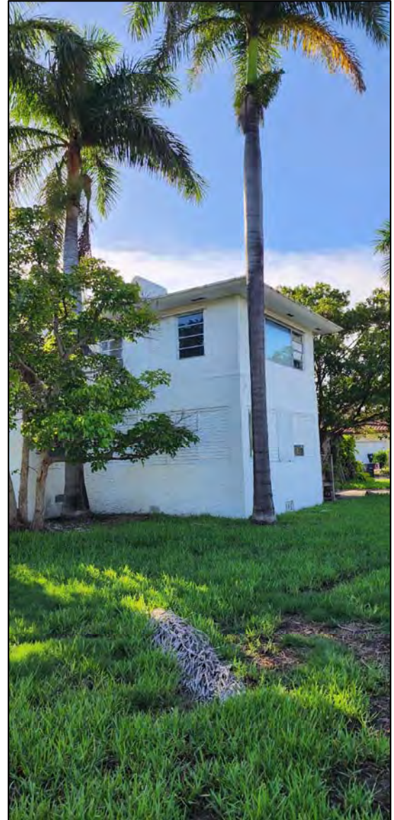
SOUTH-WEST CORNER OF THE HOUSE ( TWO STORY PORTION)
