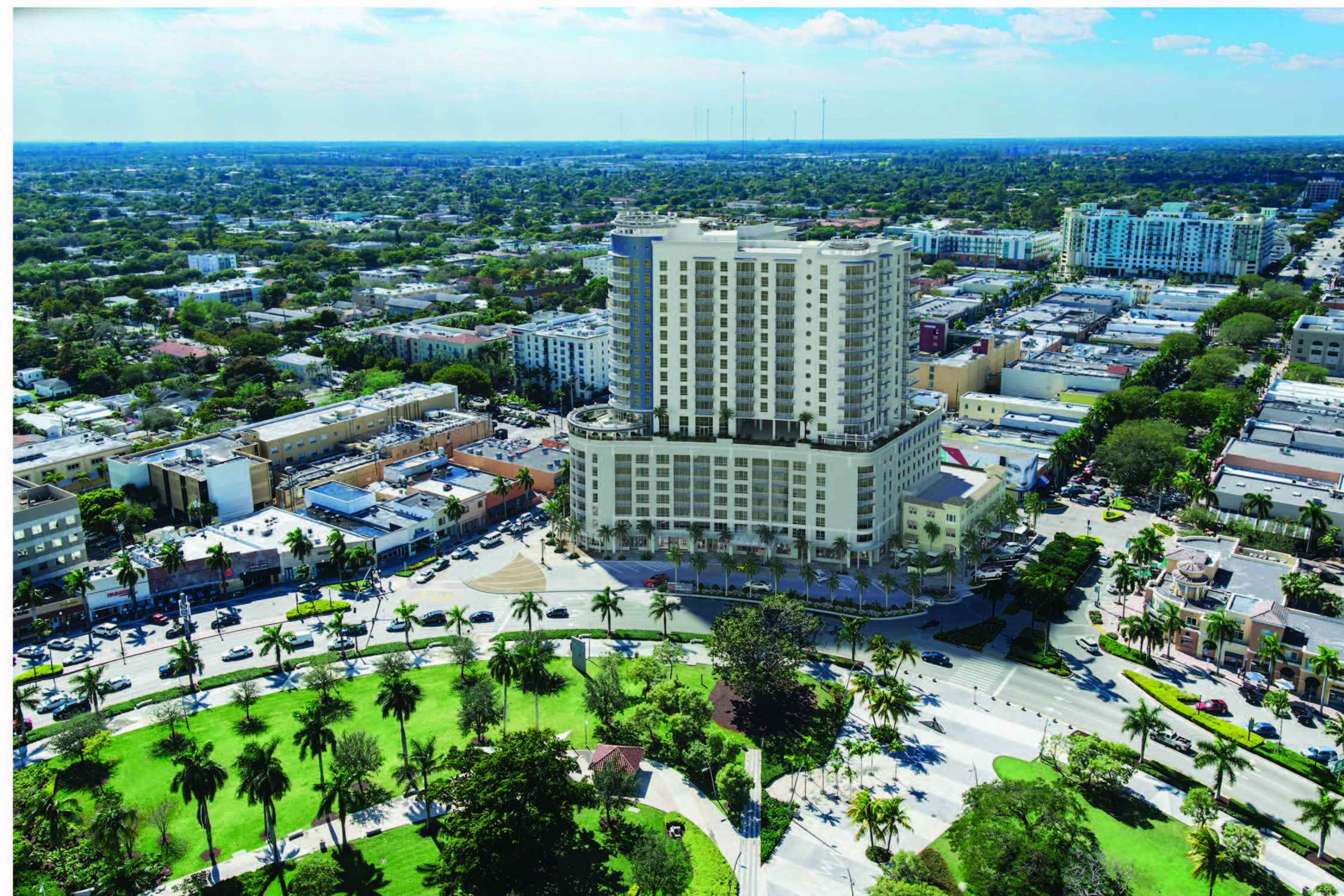
N YOUNG CIRCLE AERIAL VIEW
