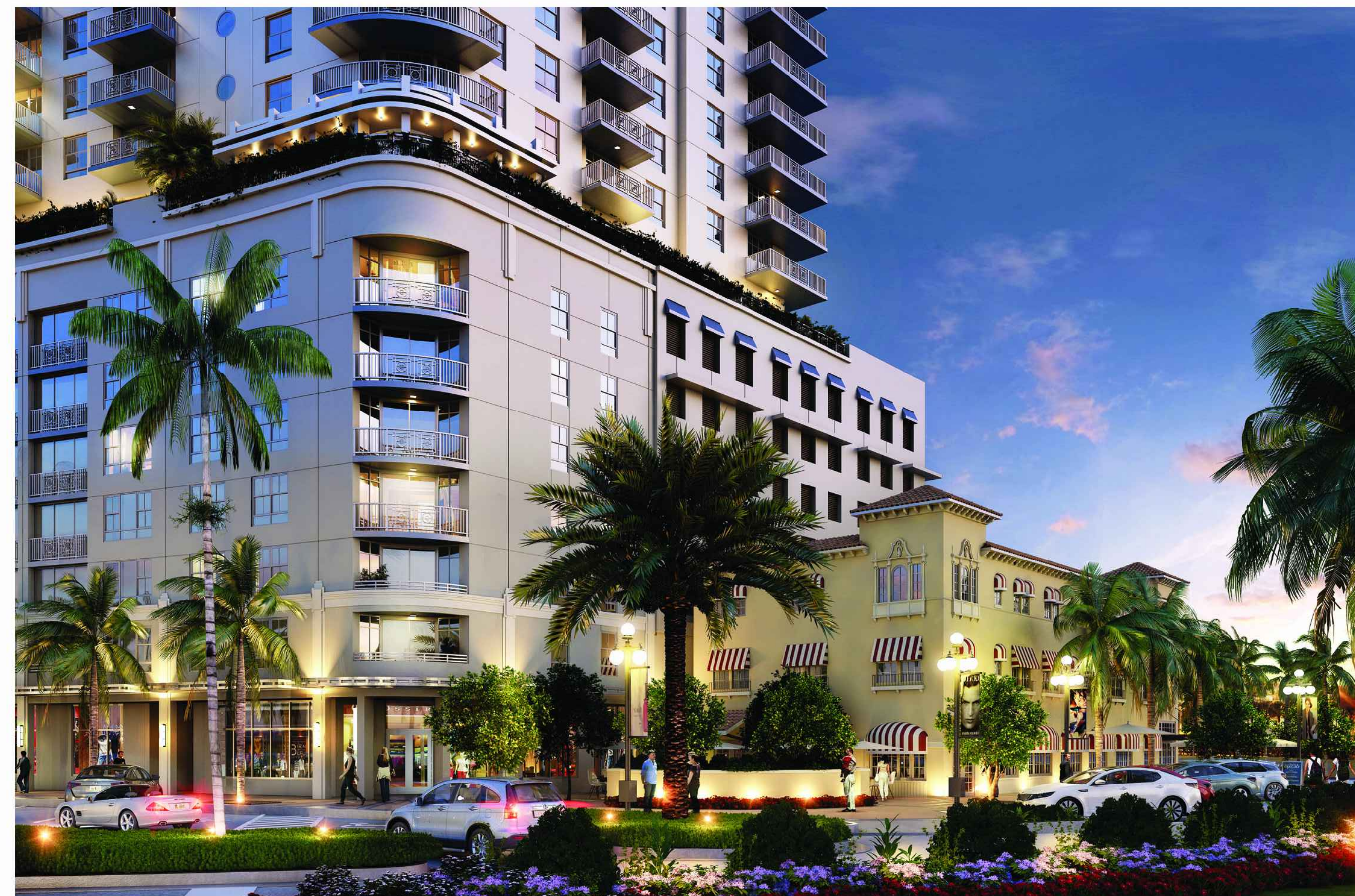
NORTH EAST ELEVATION - HOLLYWOOD BLVD.
