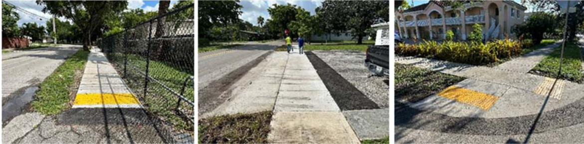
ADA ramps and sidewalks placement is substantially complete
