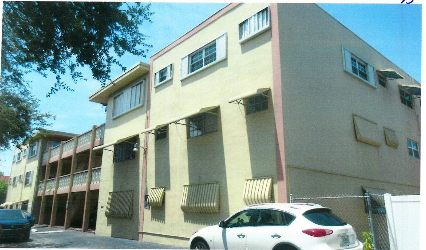
These five photo pages are a partial overview of the exterior surfaces of one three story 24 unit building known as BARCLAY ARMS CONDOMINIUM ASSOC., INC., 1943 Monroe St., Hollywood, Florida 33020.
