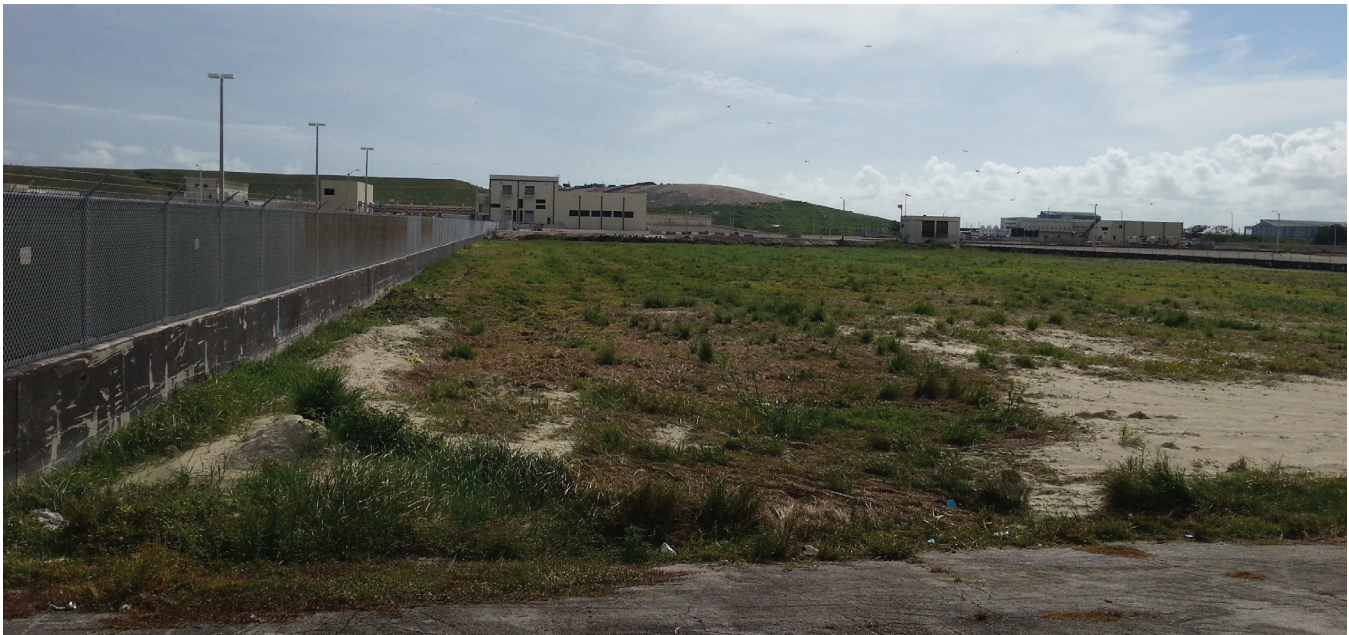
The new headworks building site will maximize the use of existing land available on the plant site.
