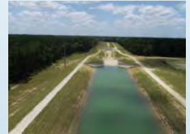
Coastal Water Authority Luce Bayou Inter-Basin Canal
