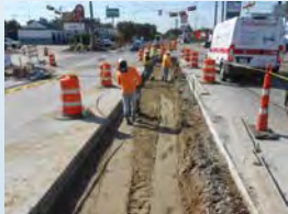
Upper Kirby Redevelopment Authority Drainage Program
