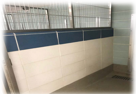
Figure 19 – Kennel Side and Sloped Floor
