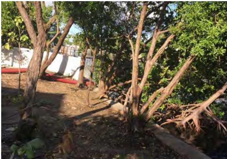
Figure 1 – Existing Seawall at 7220 Rue Notre Dame Rd.
