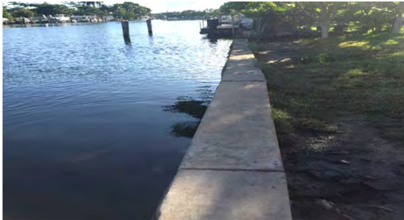
Figure 1 – Seawall along Trouville Esplanade on Normandy Island
