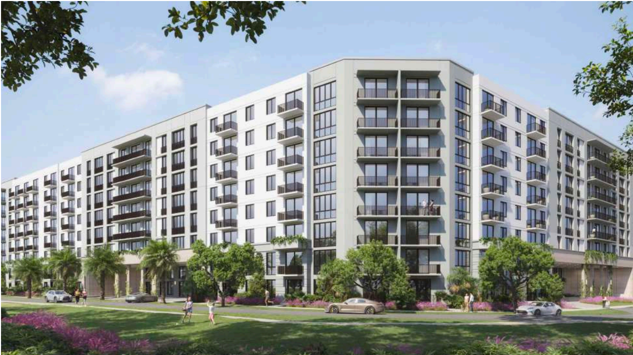
Façade Articulation: Building façades should incorporate a combination of vertical and horizontal articulation techniques to avoid visual monotony and enhance architectural expression. Variation in depth, texture, and material should be used to provide a dynamic and pedestrian-scaled environment.
