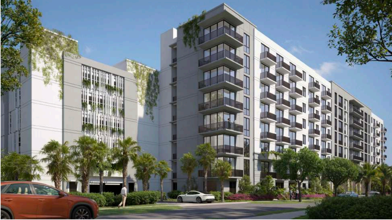
Architectural Expression: Facades should incorporate design elements that visually segment the building mass, such as horizontal score lines, contrasting base treatments with accentuated reveals, and alternating vertical color patterns to enhance architectural interest and definition.
