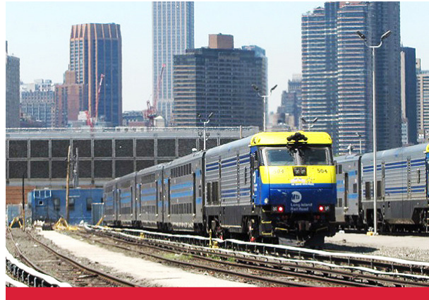
Figure C.3-2. The Long Island City (LIC) Yard. LIRR implemented restoration (recovery), integrated mitigation/resiliency, and stand-alone mitigation elements at the LIC Yard as a result of significant flooding and damage from a storm surge caused by Superstorm Sandy. Gannett Fleming is providing environmental mitigation and improvements to “harden” the area against future storm events while maintaining continuous operations in the LIC Yard. These improvements include the installation of a flood wall and flood gates around the perimeter of the yard to mitigate future storm surge flooding and damage.
