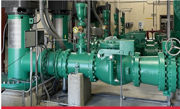
Figure C.4-2. Hopewell WTP Pump Station. To provide the existing WTP with ultraviolet (UV) disinfection treatment, advanced oxidation potential treatment for tastes and odors, replacement of their 100-year-old industrial pumping station, and replace and add chemical systems, Gannett Fleming, as part of a team, provided design-build services for improvements to VAW's WTP.
