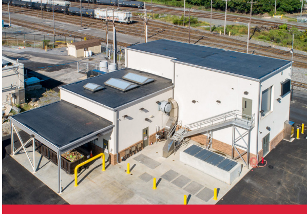
Figure E.7-3: DELCORA PS-6. Gannett Fleming served as engineer of record for this project and designed PS-6 using BIM/Revit software to replace the existing EPS-1 and to provide a pumping station with the required 28 mgd capacity influent from the collection system to meet Consent Decree Revit Design for Defense Distribution stipulations.
