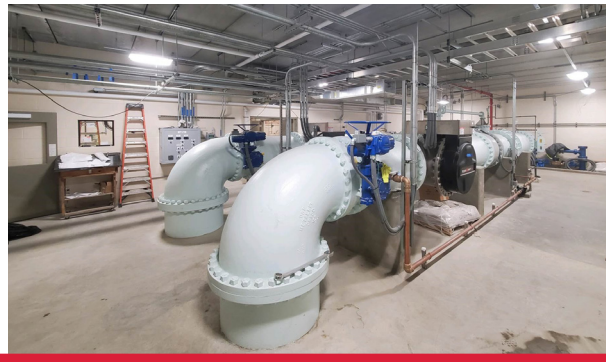
Figure C.4-2. Hopewell WTP Pump Station. To provide the existing WTP with ultraviolet (UV) disinfection treatment, advanced oxidation potential treatment for tastes and odors, replacement of their 100-year-old industrial pumping station, and replace and add chemical systems, Gannett Fleming, as part of a team, provided design-build services for improvements to VAW's WTP.
