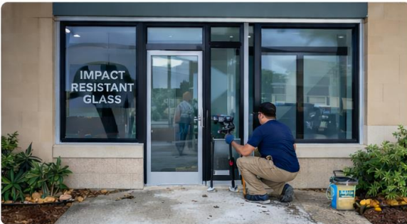
Window & Door Replacement
