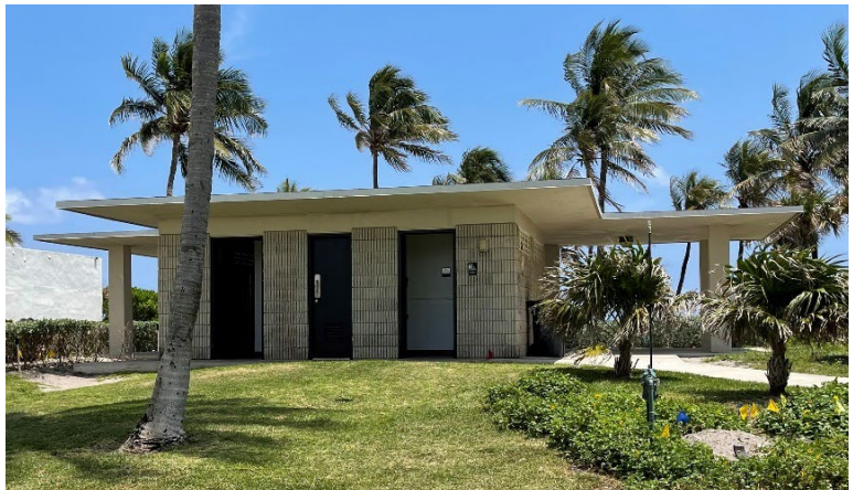
Keating Park Pavilion Looking West
