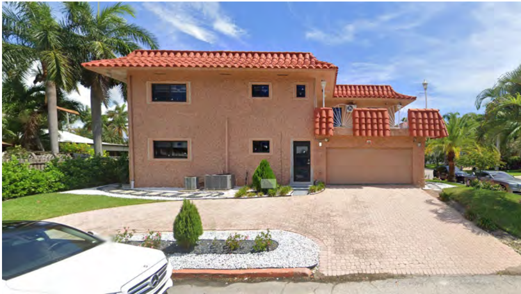
900 S. Southlake Drive (southwest)
