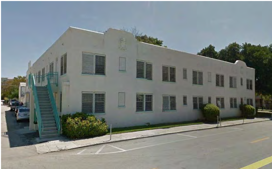
1957 Jackson Street (Southeast corner from site)
