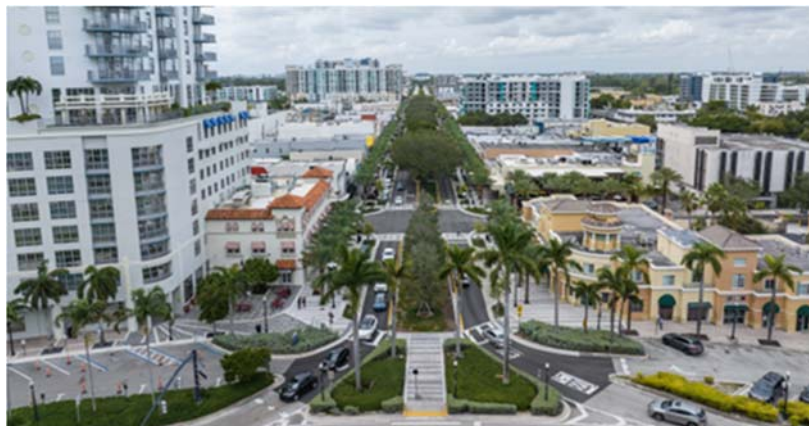
Aerial view of completed streetscape
