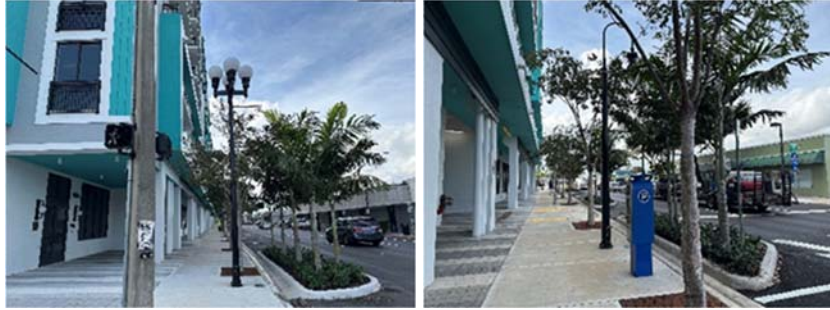
Installation of new light poles and fixtures
