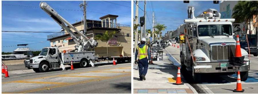
AT&T connection and overhead wire removal
