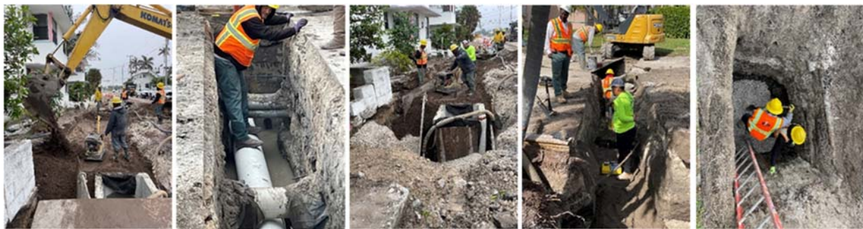
Excavation, trenching, existing conditions evaluation (Harrison and Van Buren Streets)
