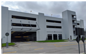
FAU GARAGE III
