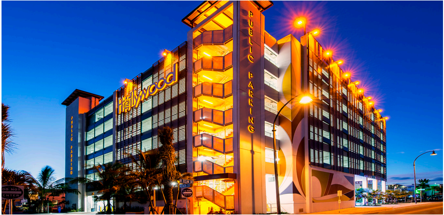
HOLLYWOOD NEBRASKA ST. PARKING GARAGE $13.1 MILLION
