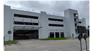
FAU GARAGE III
