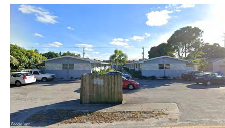
E STREET VIEW PHOTO 2330 POLK STREET N.T.S.
