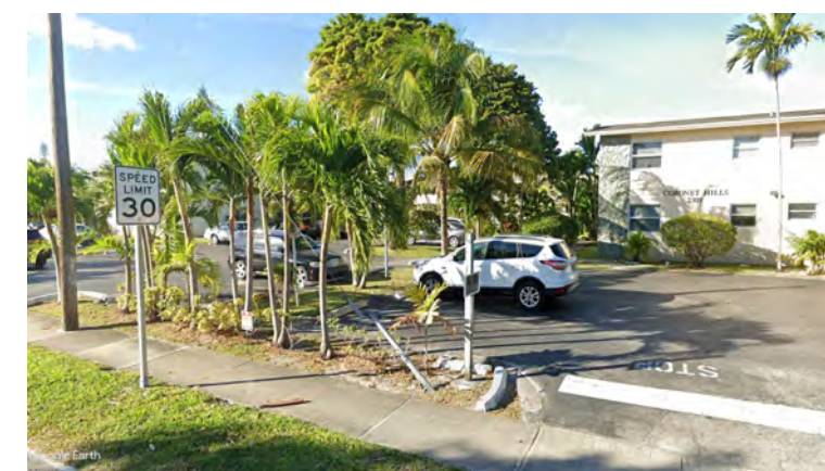
C STREET VIEW PHOTO 2320 POLK STREET N.T.S.
