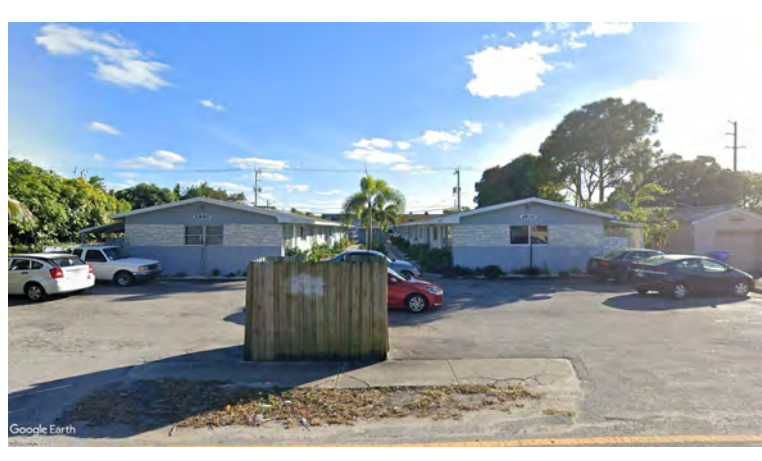
E STREET VIEW PHOTO 2330 POLK STREET N.T.S.
