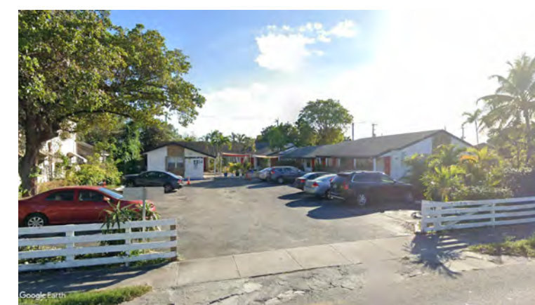
D STREET VIEW PHOTO 2314 POLK STREET N.T.S.
