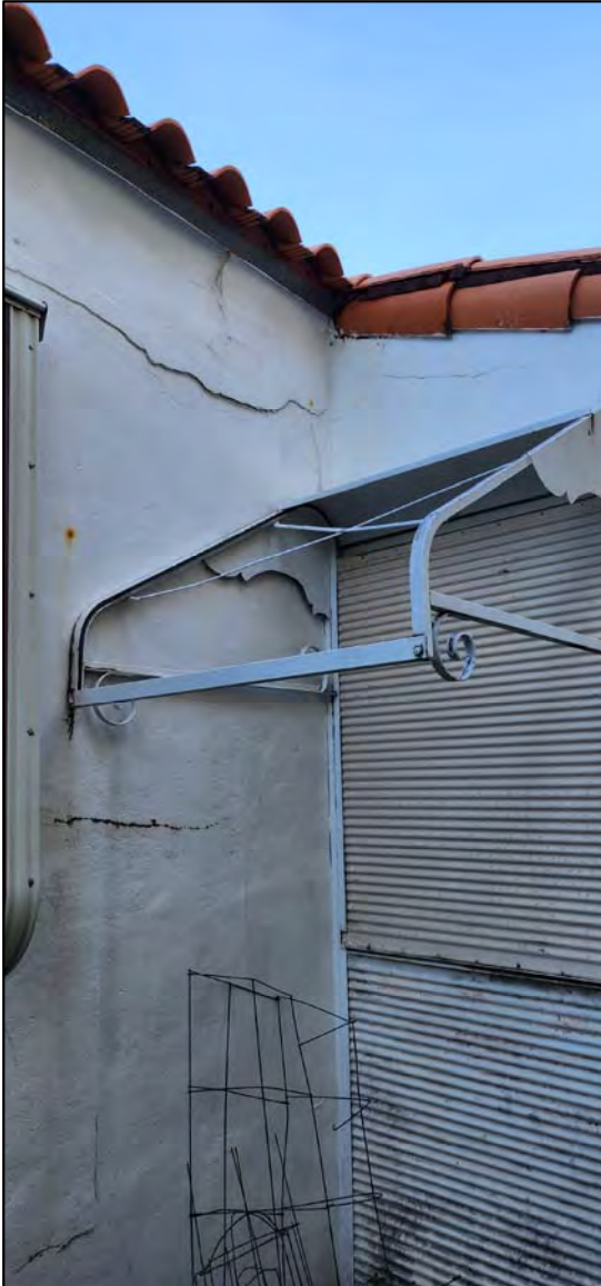
WALL CRACKS AND SPALLED AND CRACKED ROOF BEAM
