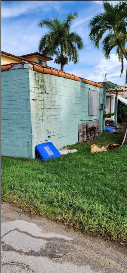
STEP DOWN CRACK ON EXTERIOR WALL
