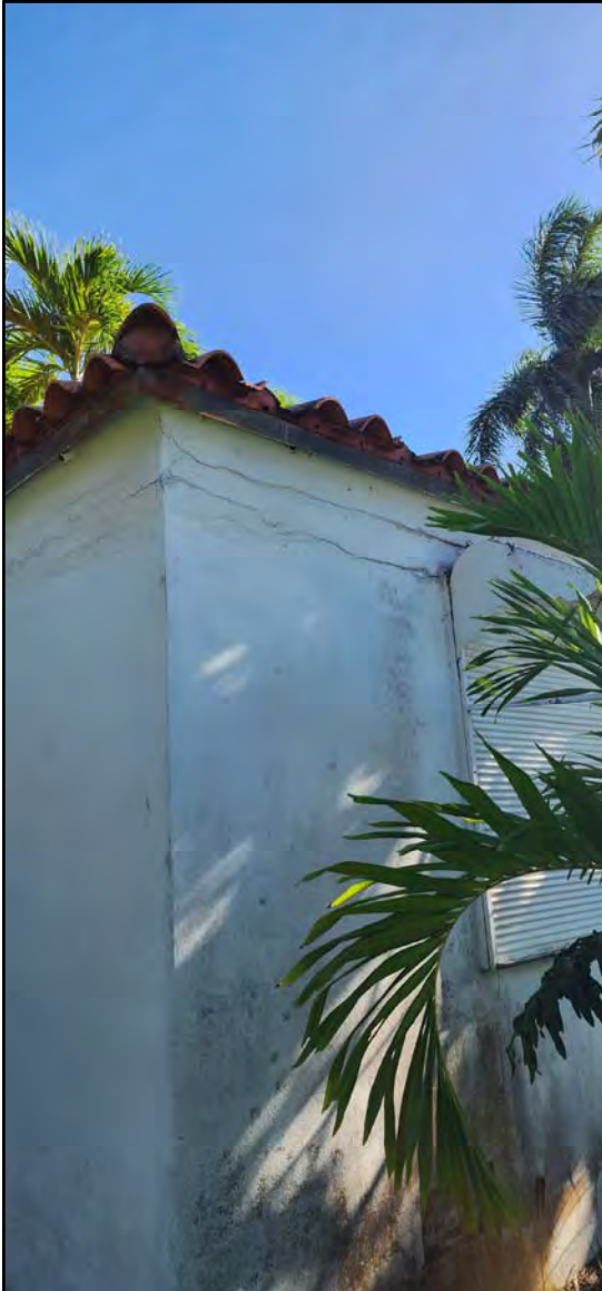
CONTINUOUS CRACK UNDER ROOF TIE BEAM
