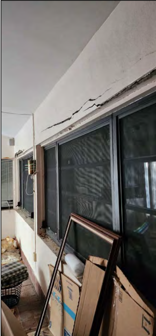
DAMAGED AND CRACKED BEAM ABOVE THE WINDOW
