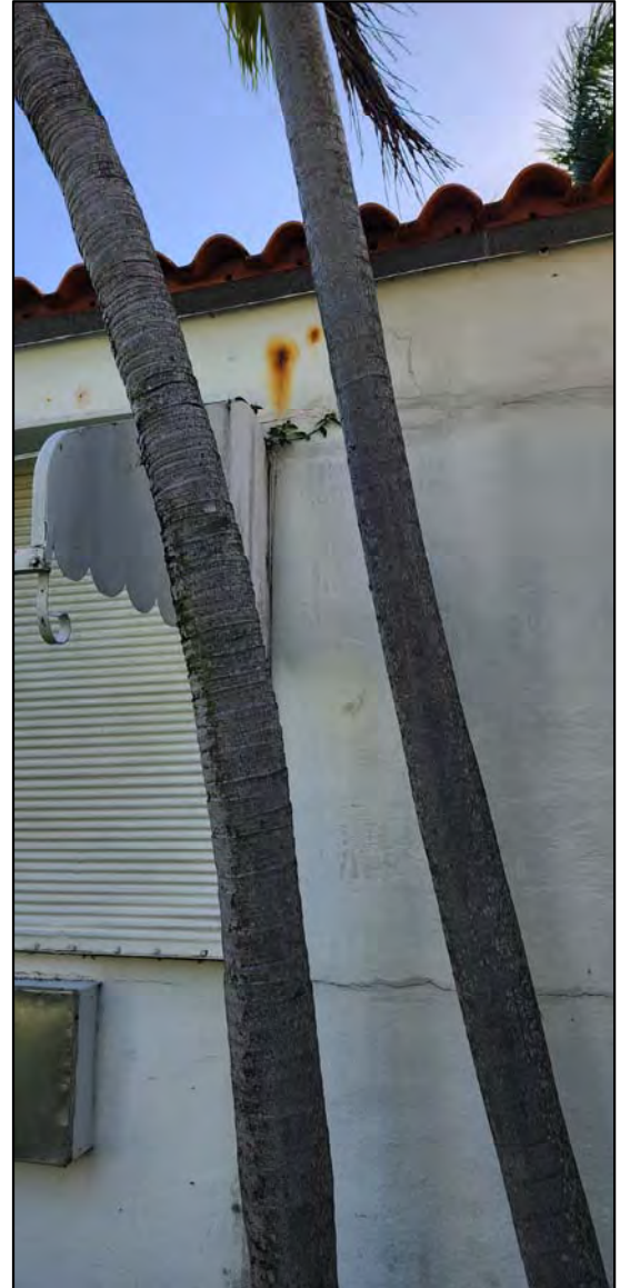
ROOF BEAM, RUST BLEEDING AND WALL CRACK
