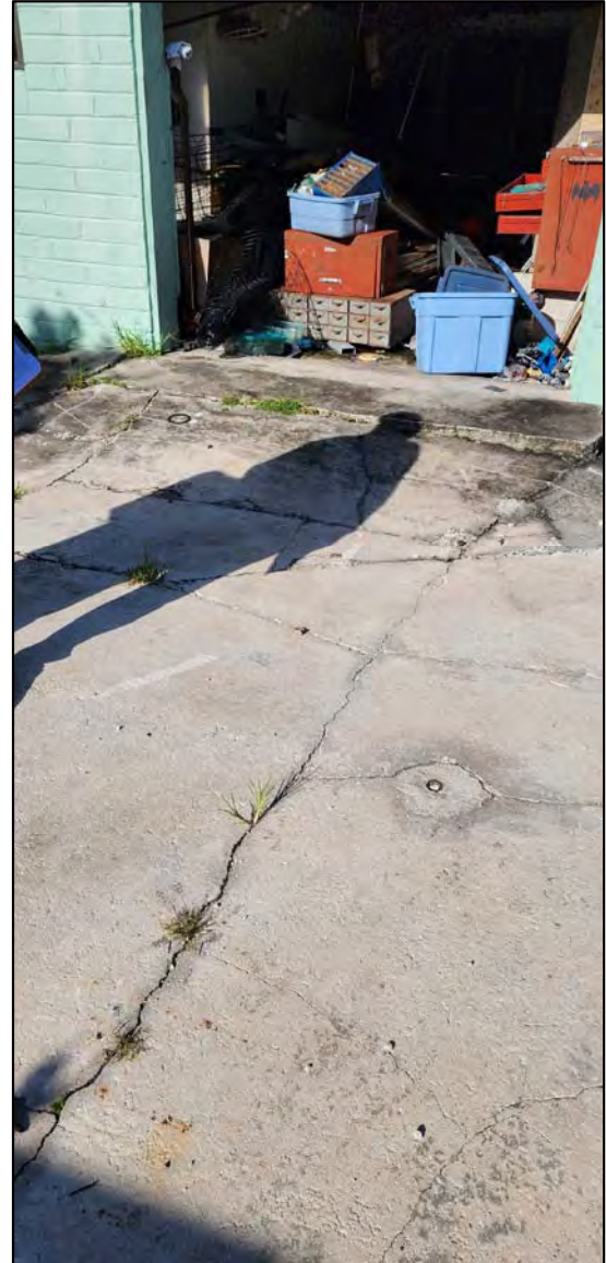
WEST ENTRANCE TO DETACHED STRUCTURE WITH CRACKED CONCRETE SLAB
