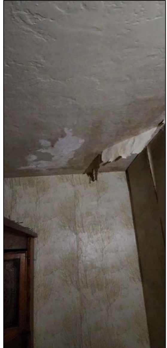
MOISTURE INTRUSION AND DAMAGED CEILING
