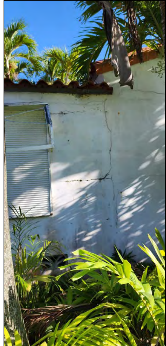
EXTERIOR HORIZONTAL AND VERTICAL CRACKS ADJACENT TO THE WINDOW
