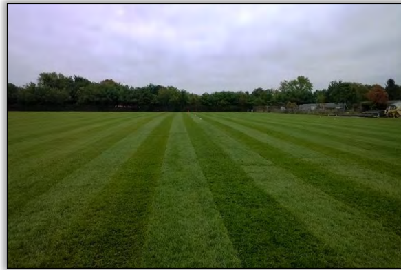
Completed Site Restoration Riverwood Park, Toms River, NJ
