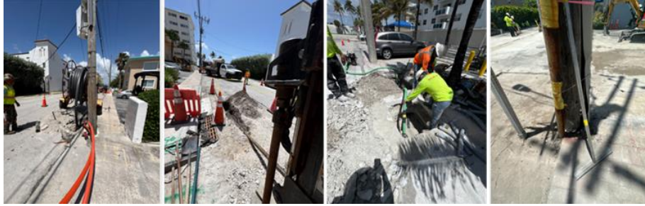
Undergrounding and electrical infrastructure installation, private property conduit runs
