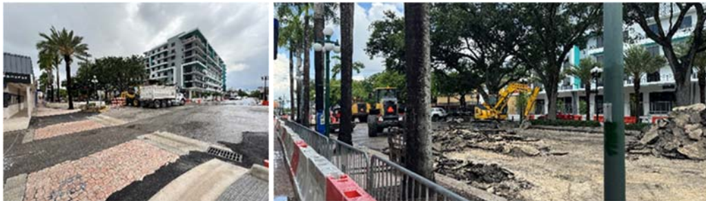
S. Hollywood Boulevard, 20 th & 21 st Ave: Demo of existing roadway, curb, and gutter.
