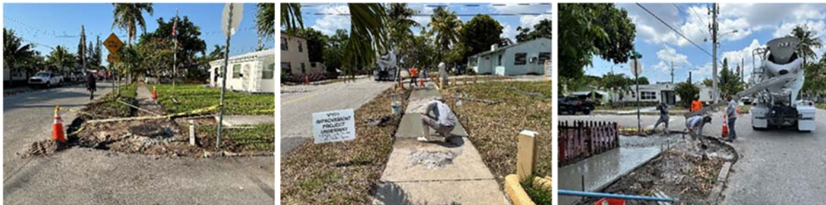
Demolition of ADA ramps and sidewalks, and placement of concrete
