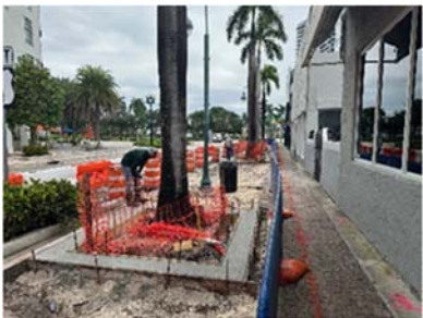
Placement of new tree pits
