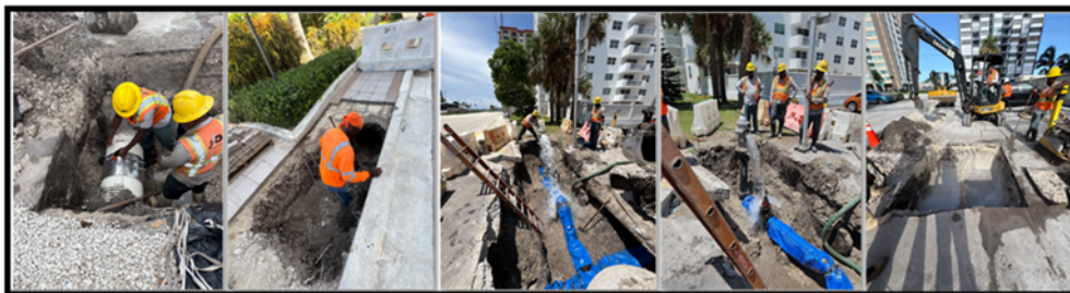
Coastal Resiliency Phase IV stormwater and fire hydrant installation.
