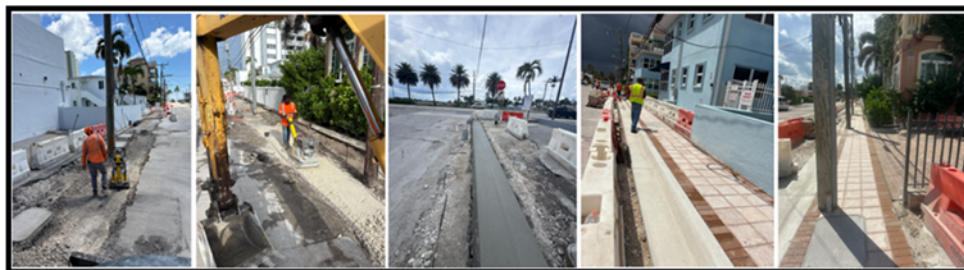
Demolition of existing south sidewalk; installation of new valley curb and hardscape Coastal Resiliency Phase IV sidewalk installation on Van Buren Street.
