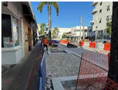
Rough grading sidewalk
