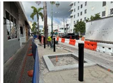
Forming bollard foundations
