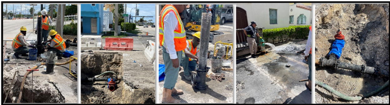
Replacement and connection of new fire hydrants.
