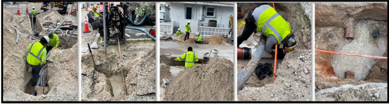
Undergrounding and electrical infrastructure installation, private property conduit runs
