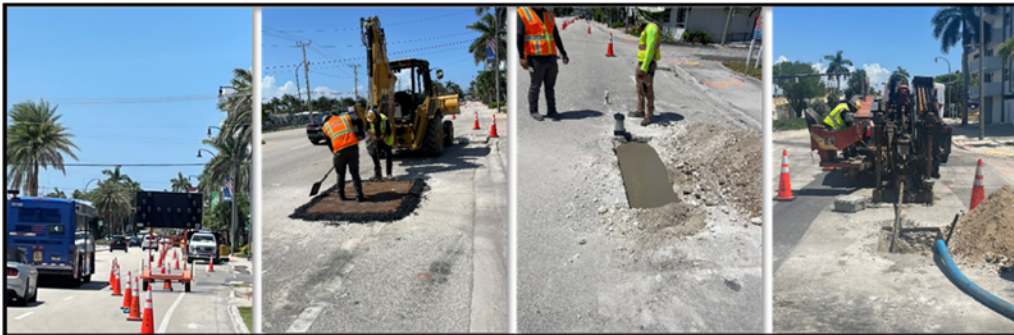
Undergrounding and electrical infrastructure installation, private property conduit runs
