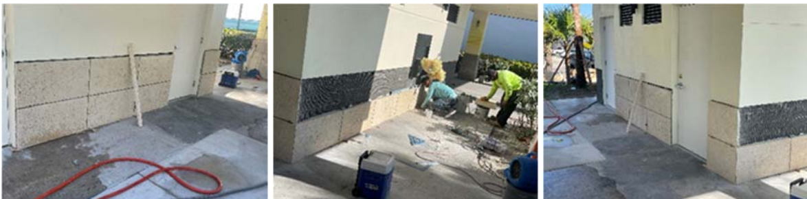
Installing the coquina cast stone on Keating Park restroom building
