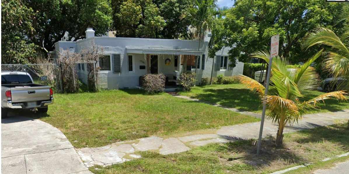
1735 Jackson Street – Subject property (view to South)
