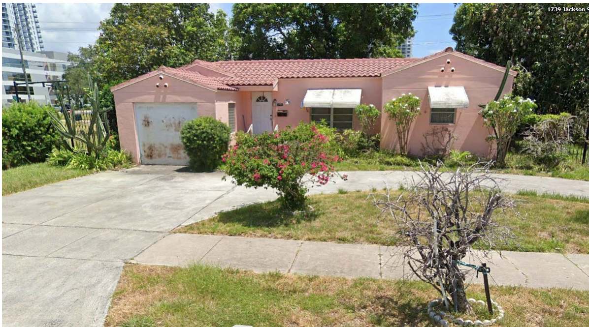
1739 Jackson Street – Subject property (view to South)
