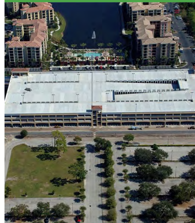
Left: Ocean Reef Club Village Parking Garage Above: Orlando Vineland Premium Outlets Parking garage
