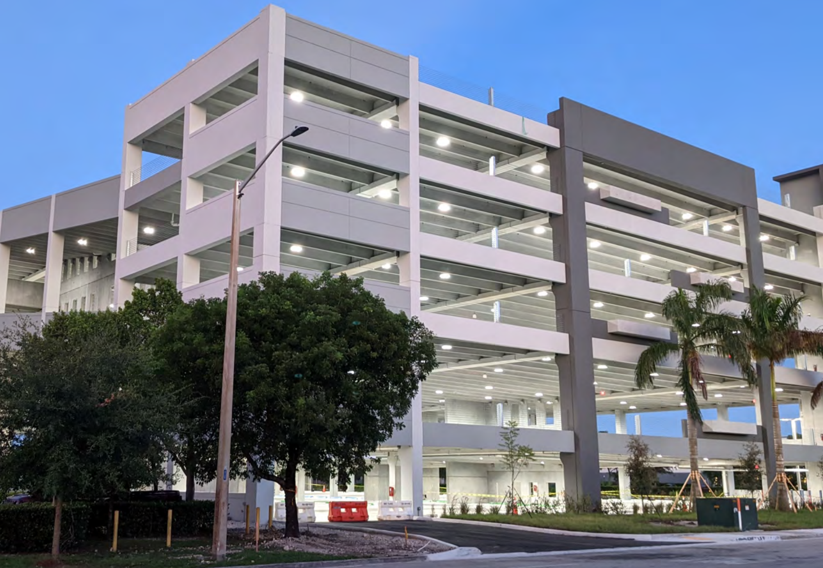
MIAMI LAKES AUTOMALL GARAGE
