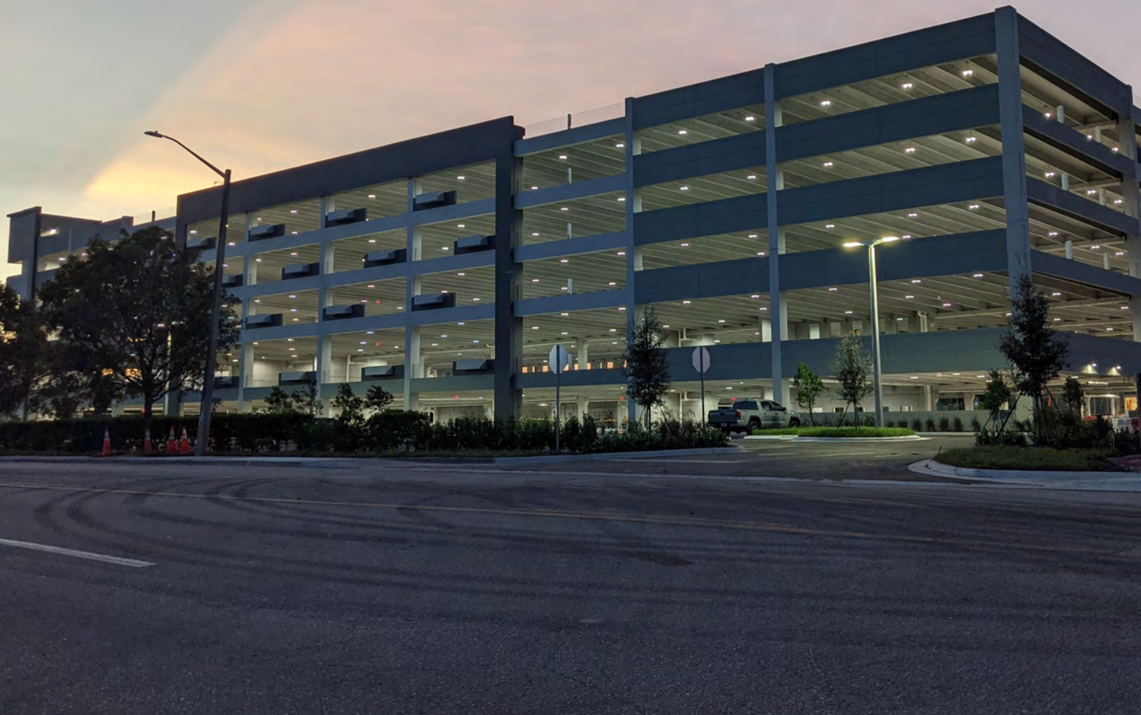
MIAMI LAKES AUTOMALL GARAGE
