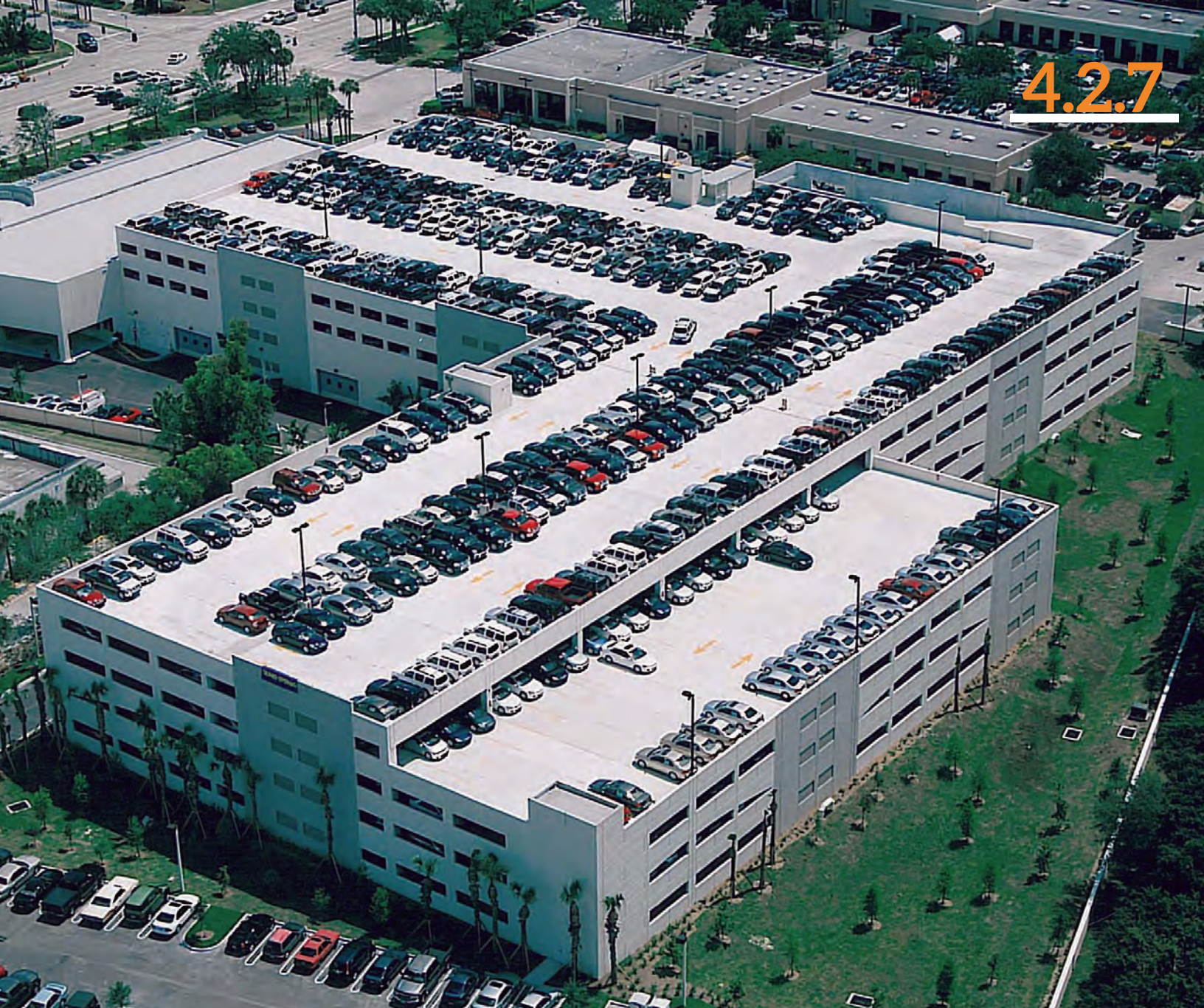
CORAL SPRINGS AUTO MALL & PARKING GARAGE
