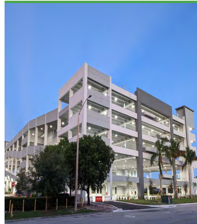
Left: Memorial Hospital DB Parking Garage Above: Miami Lakes Automall Garage
