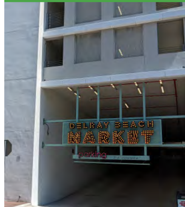
Left: City of Lake Worth Beach Downtown Parking Above: City of Delray Beach Parking & Curb Management
