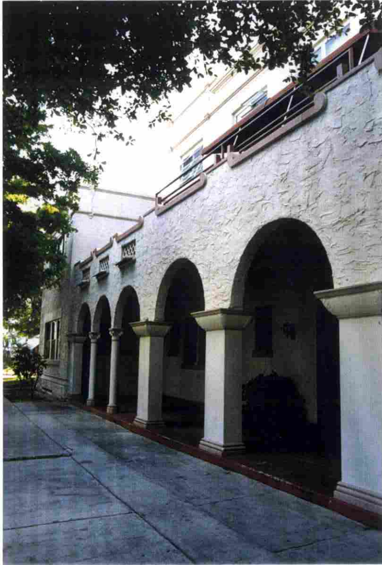
Front loggia note: Block columns
