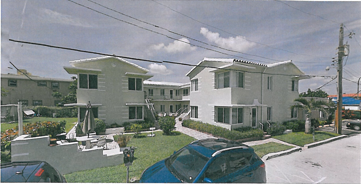
320 MCKINLET ST (south)
