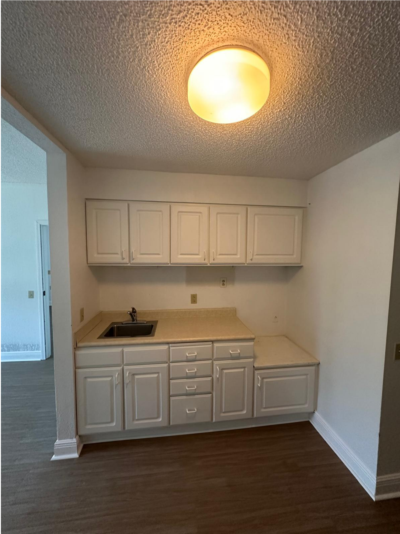
EXISTING KITCHEN ELEVATION
