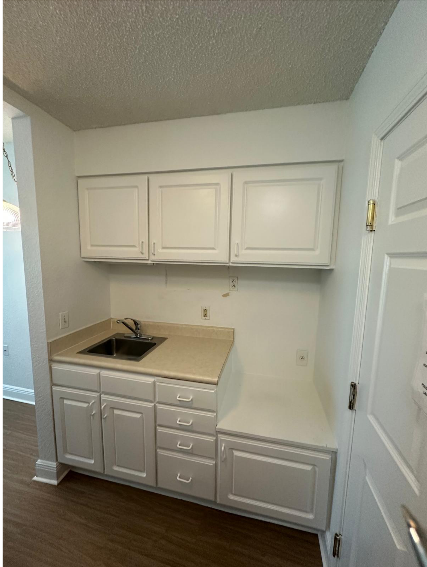
EXISTING KITCHEN ELEVATION
