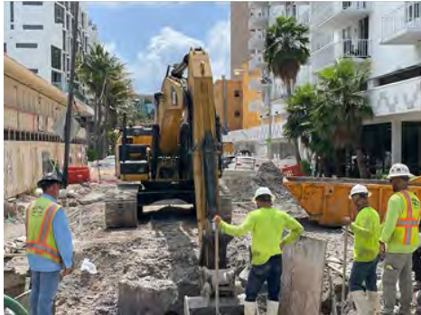
Figure 1 – Construction of stormwater culvert
