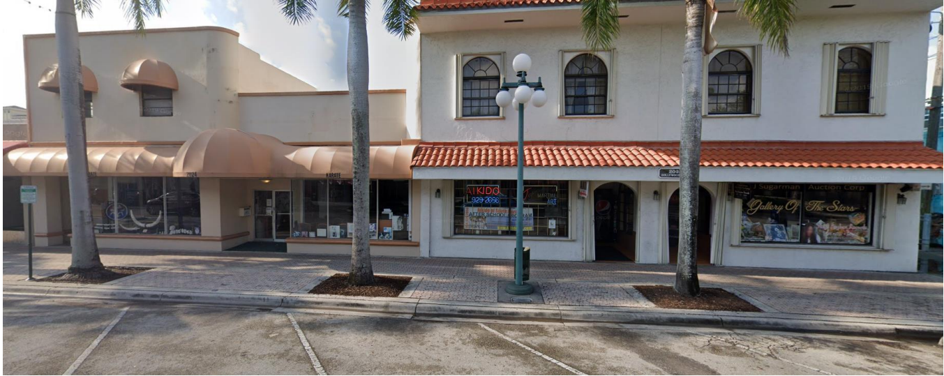
South adjacent properties
