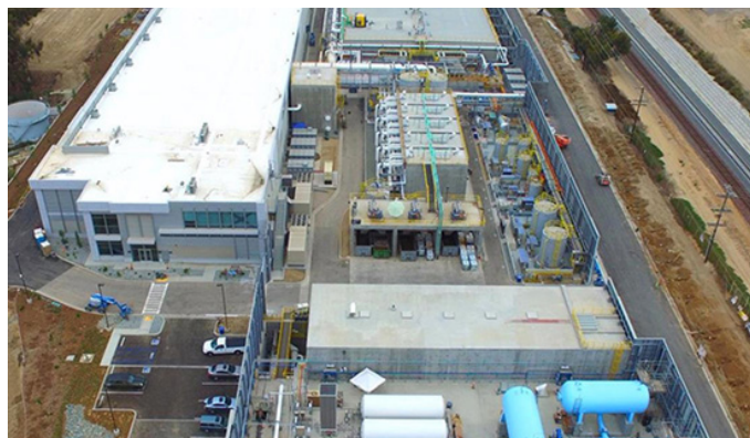
Carlsbad Desalination Plant (50 MGD) was design by Arcadis and 2017 ACEC National Grand Award Winner.
