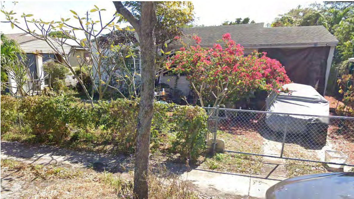
1840 Mayo Street – Subject property (view to South)
