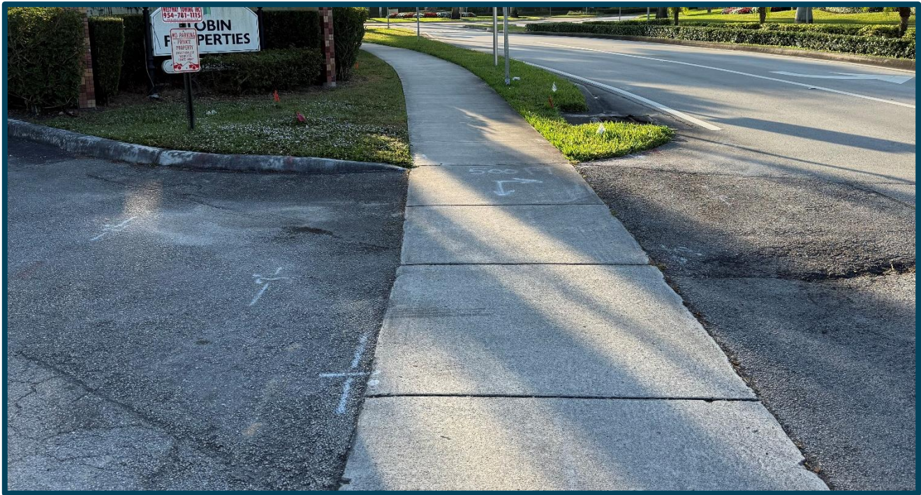
Sidewalk provided along the north side of Hillcrest Drive, south of the north project driveway (Looking south)
