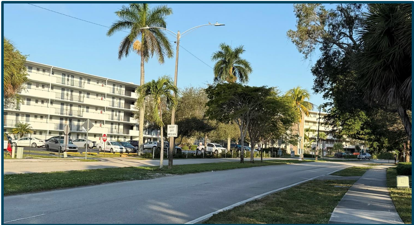
Dual-mast lighting provided within the median along Hillcrest Drive, west of Parkview Drive (Looking north)
