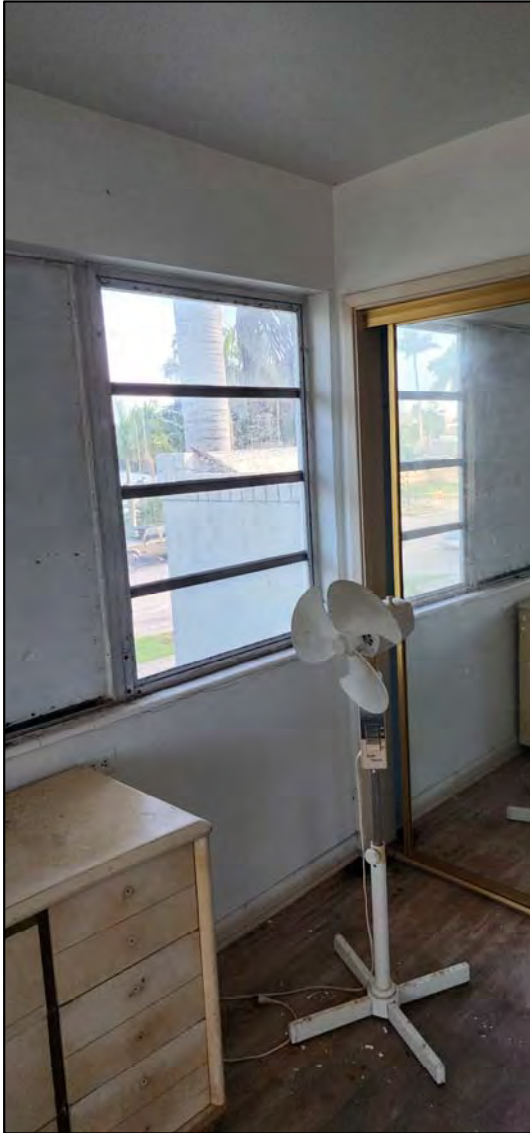
PARTIAL VIEW OF SECOND FLOOR
