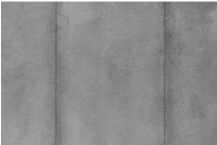
Raw Concrete Ground floor and accent walls
