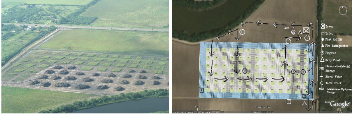
An Aerial view of a DMS used by Ceres in the past and its site layout plan.
