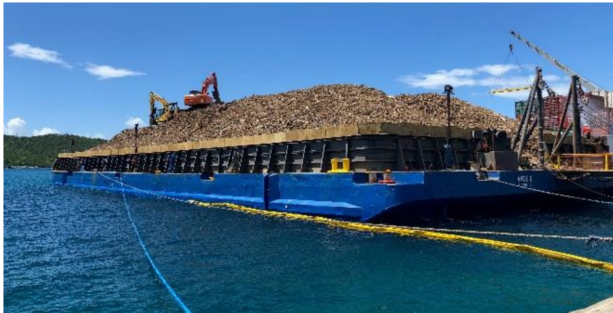
Ceres Off-Island Disposal of Shredded C&D Debris Shipment Headed for Texas
