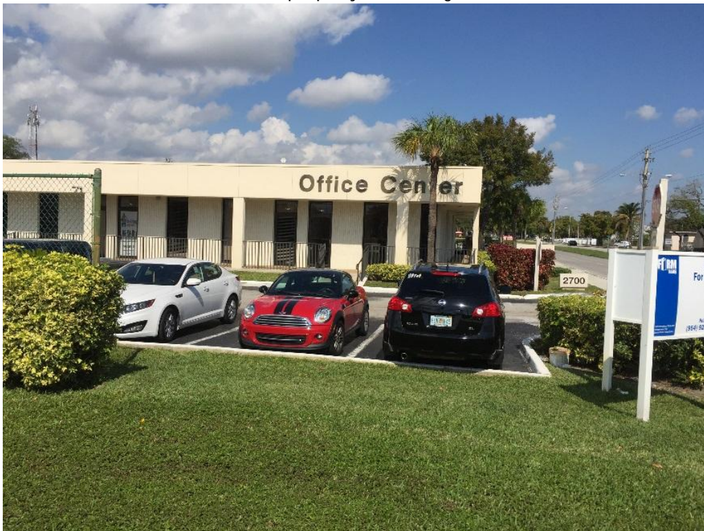
2. Northeast corner of North property line, facing north.
