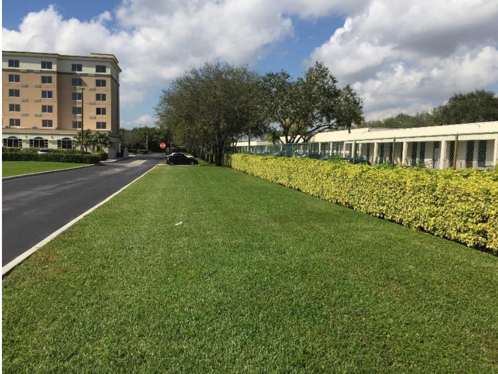
1. Northeast corner of North property line, facing westward.
