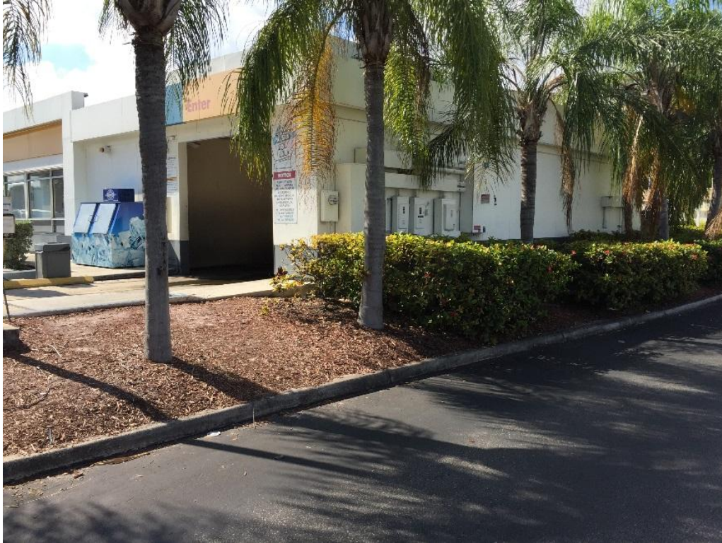
9. Property to south (existing car wash)
