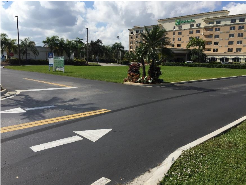
4. Northeast corner, facing southwest
