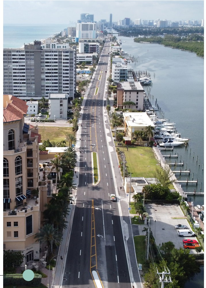
TETRA TECH IS ASSISTING THE CITY TO MEET ITS INFRASTRUCTURE NEEDS DUE TO REDEVELOPMENT ON HOLLYWOOD BEACH
